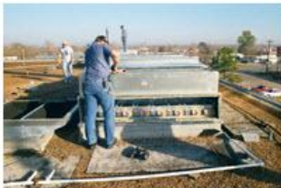
The new curb and dampers are fitted to the existing curb.
